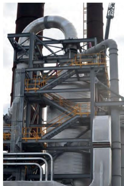
**The thermal oxidizer in the new air emissions control system at Orion’s plant in Belpre, Ohio - Thermal oxidizers are devices that control emissions by combusting them**
