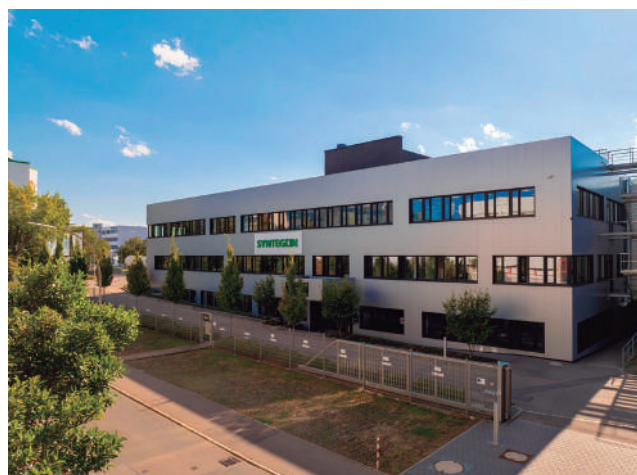
Following the move from Waiblingen, Syntegon has opened its new OSD Customer Center in Fellbach
